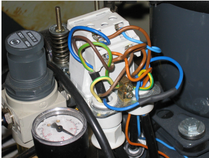
Connected wires on main switch with zero relay. Fig 2
